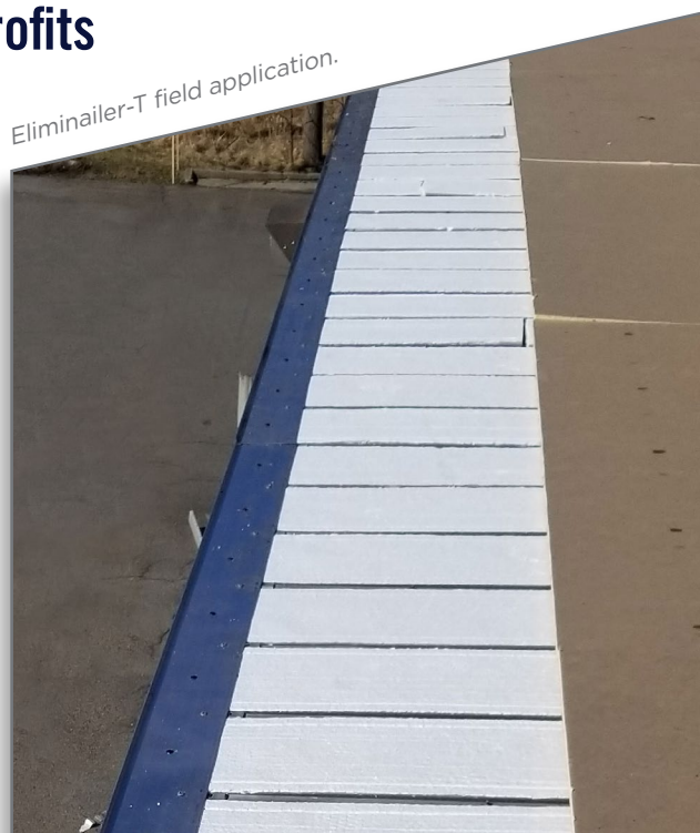
Eliminailer-T shown on flute-filled application featuring Anchor-Tite Drip Edge.
